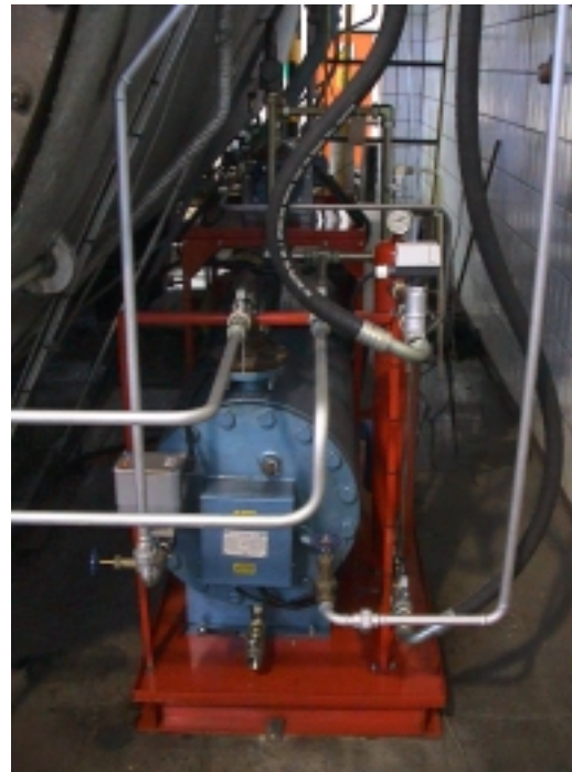
Pump skid incorporating Steam Electric heater and Autoflame controls
