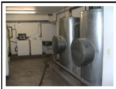
After: 1500L hot water storage and space for an in house laundry.
