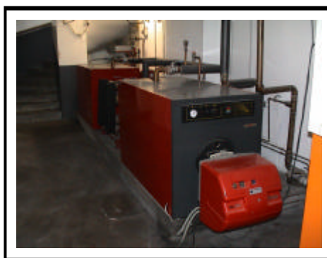
2 x 220 kW diesel fired boilers
