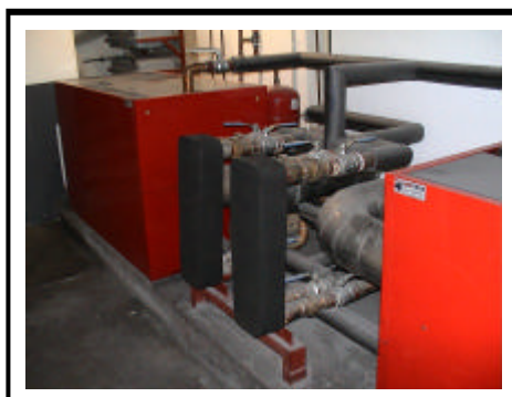
Heat exchangers to ensure constant 60°C hot water
