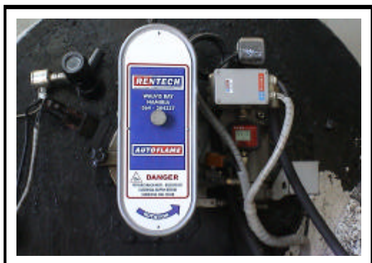
Burner with Autoflame controls
