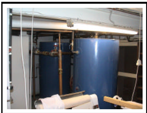
2 x 500L Hot Water Storage Tanks
