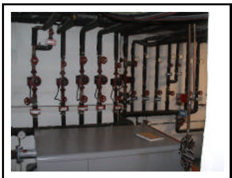
7 Hot Water Circulating Pumps
