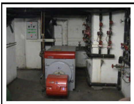
New 180 kW Diesel Ferroli Boiler
