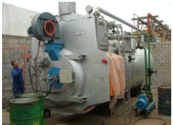
Boiler after refit and conversion to Autoflame
